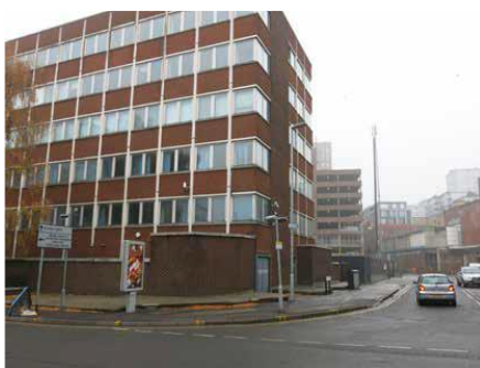
View of the Site from Greyfriars Road
