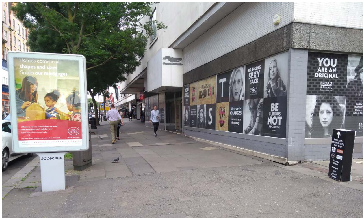
Existing Oxford Road frontage looking east
