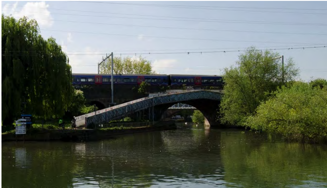
Figure 3.5: Stepped Horseshoe Bridge
