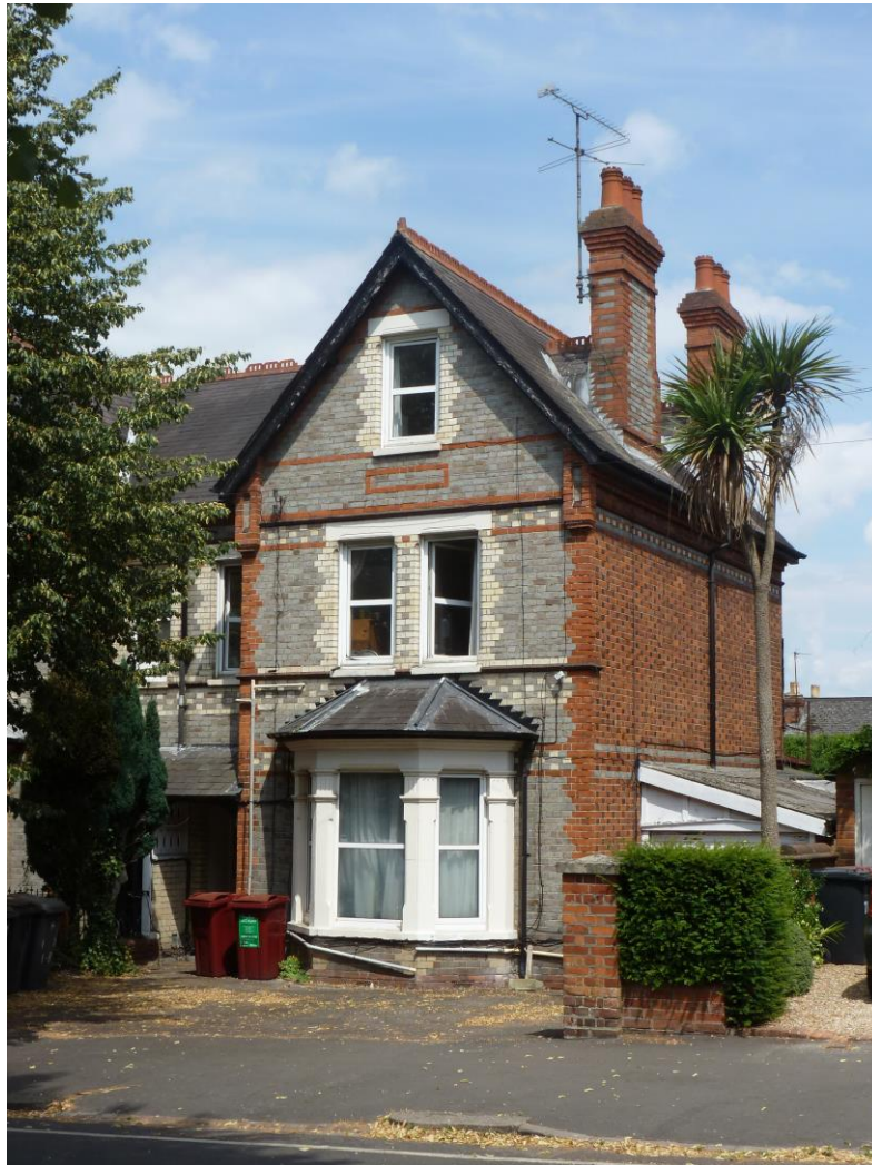
Fig.1: View of 71 Alexandra Road from the street.
