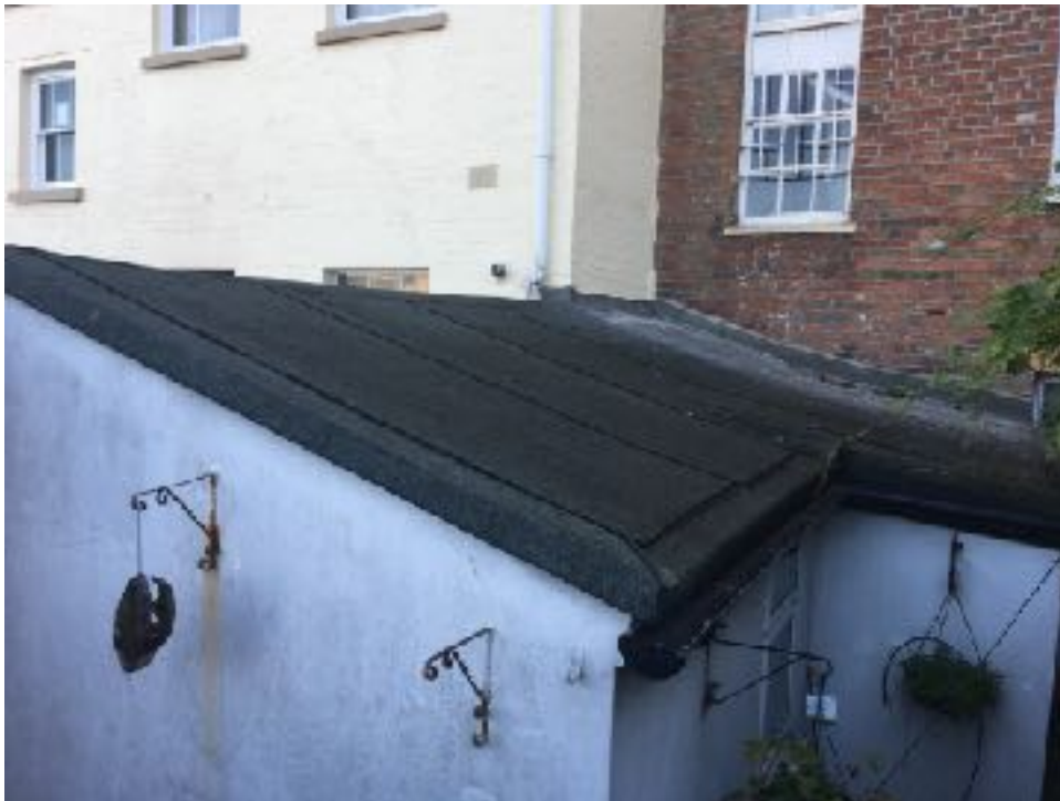
Figure 1 Flat roof over rear extension
