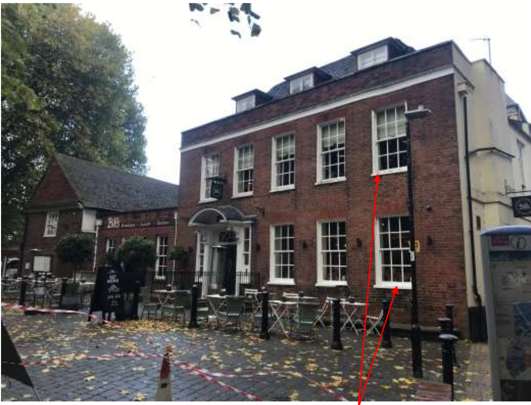
Window planters located on ground and first floor windows
