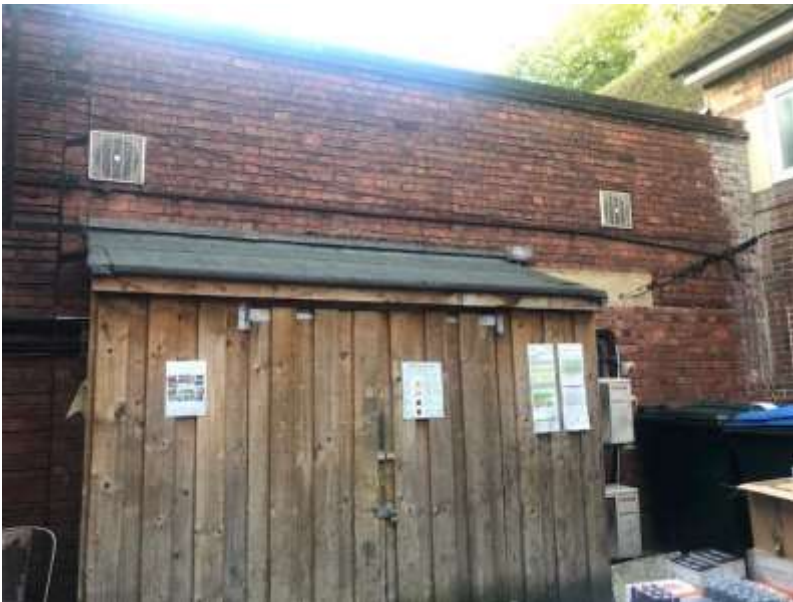
Photograph of north wall of 1931 extension. Proposed kitchen extension abuts this wall.
