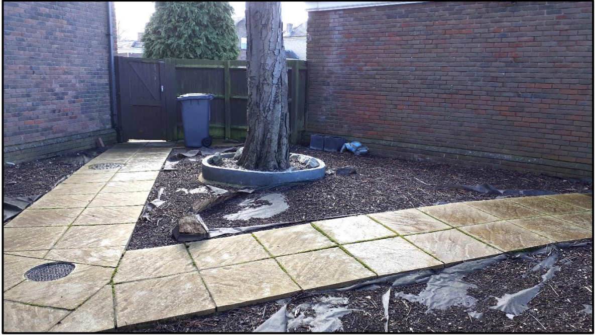
Photograph 5. Close up of base of T1 showing existing layout of hard surfacing, paving and unsurfaced ground, and proximity of the tree to main dwelling elevations and garage building. The Lawson cypress in the background is in the front garden of 11 Devonshire Park and provides some screening of the tree from certain views. Viewed looking towards the south-west.
