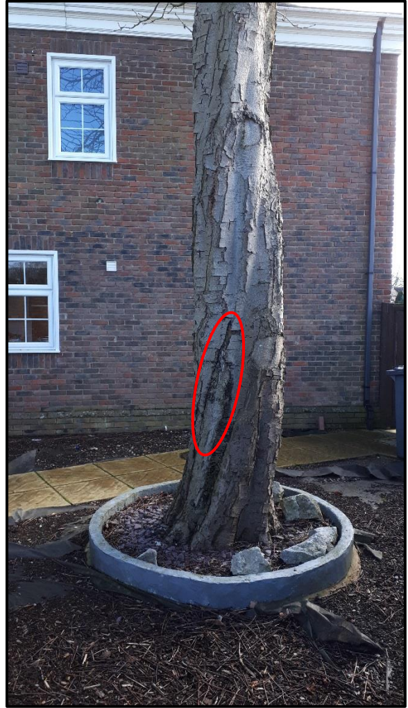
Photograph 2. Close-up of the main stem of T1 showing minor area of bark lesion to the north-west. Viewed looking towards the south.
