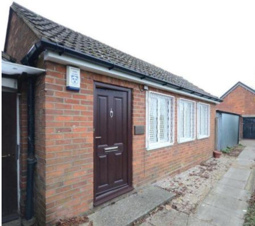
Fig 3: East elevation of the office building
