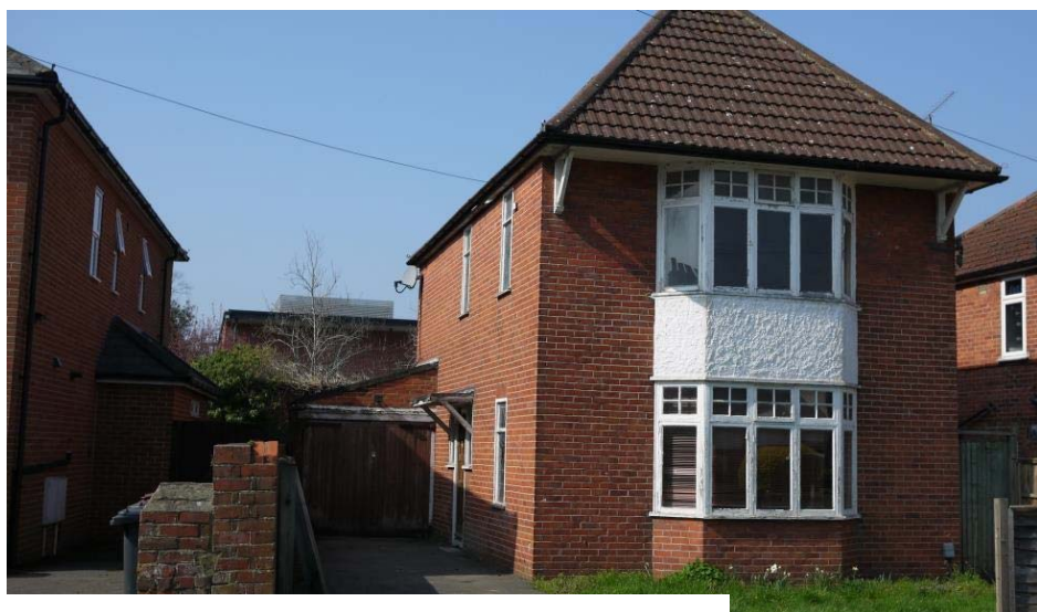
“Two storey side extension not present in the photograph.
