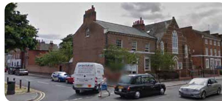
Oxford Road / Howard Street Corner
