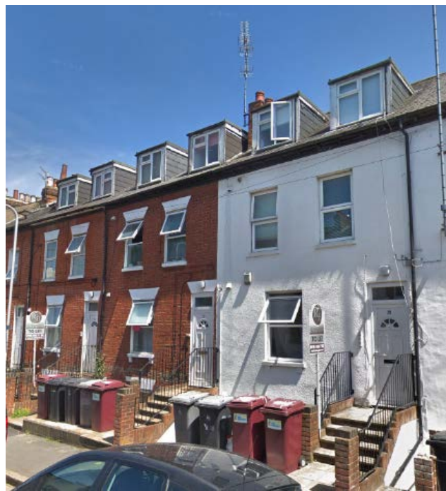
Photograph 2: Dormers at Zinzan Street (Google Earth)
