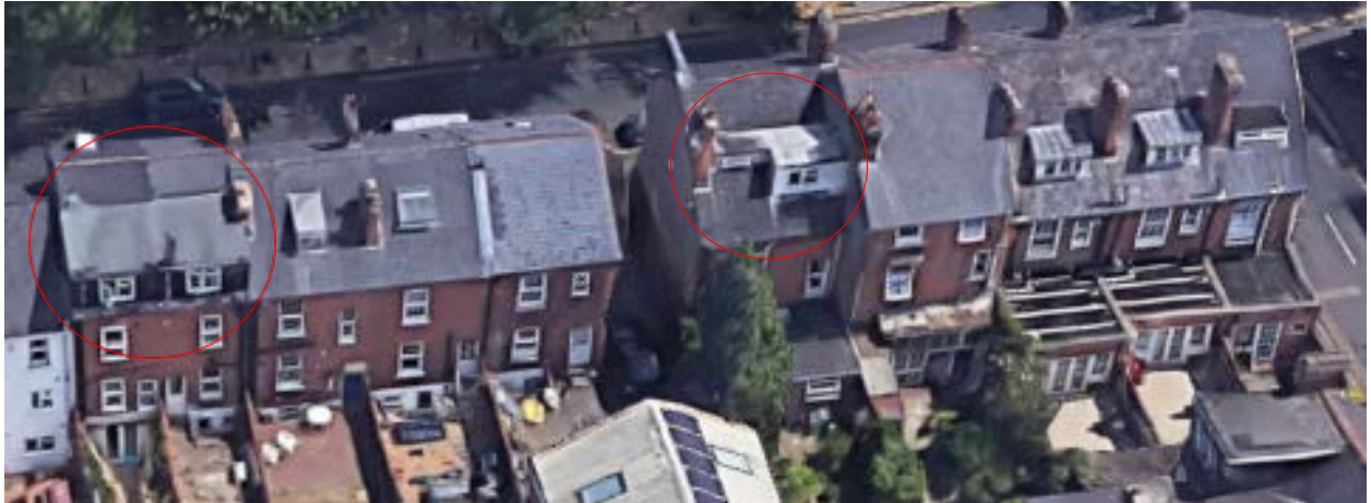
Photograph 3: Large flat roof rear dormers at Howard Street (Google Earth)
