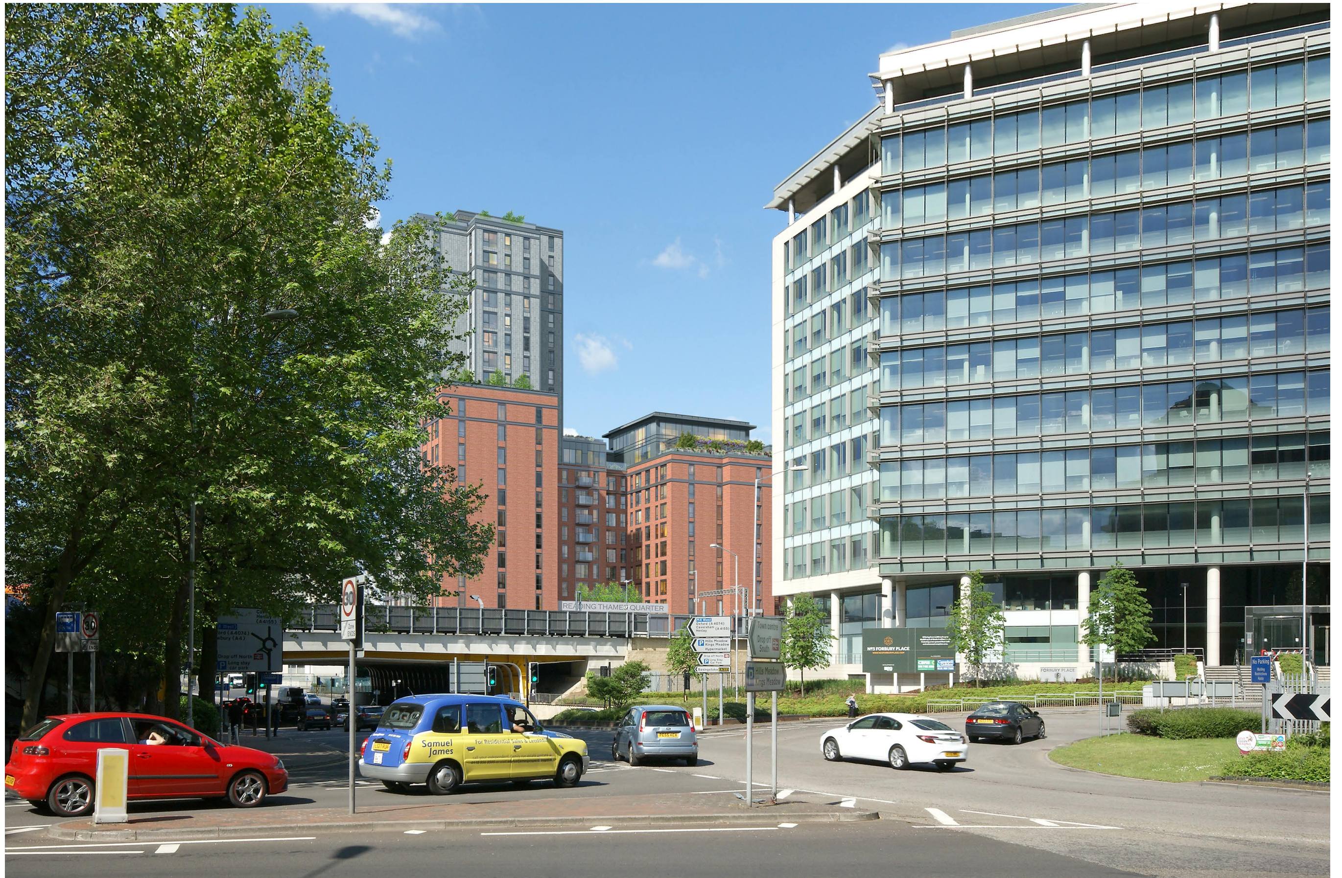
AVR view north north-east from Forbury Road
