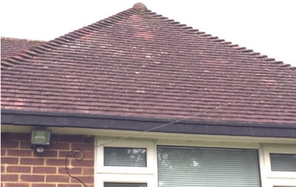
Figure 8. Clay tiles sitting flush on roof top at the northern end.
