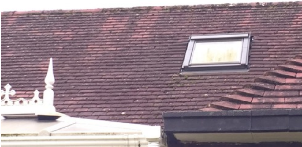
Figure 9. Clay tiles sitting flush on the east-facing roof.
