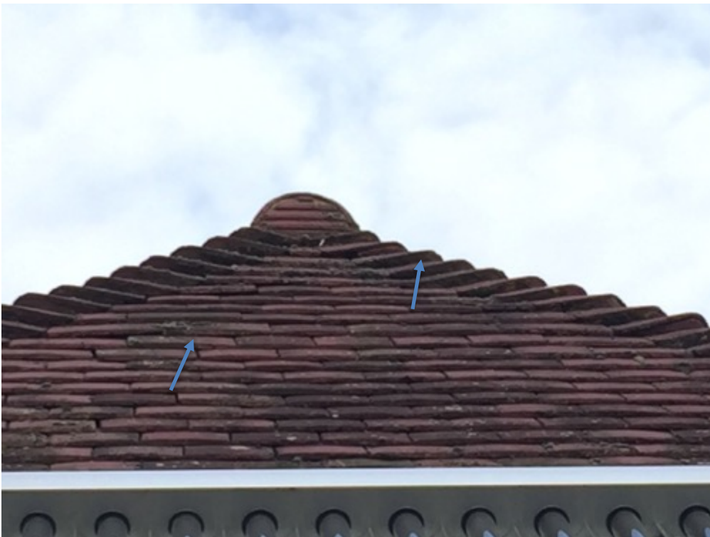
Figure 6. South facing roof with two gaps potentially suitable for crevice dwelling bats.
