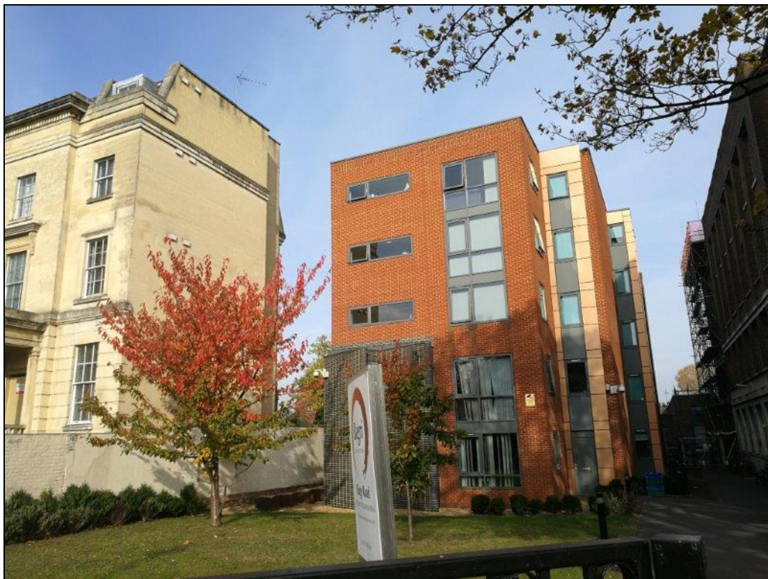
Fig. 1 – 191 Kings Road – Front Entrance
