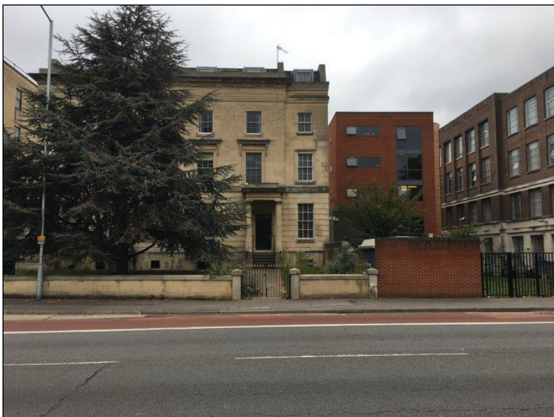
Fig. 2 – 187-189 Kings Road – Front Elevation to the left of 191 Kings Road with Reading College to the right
