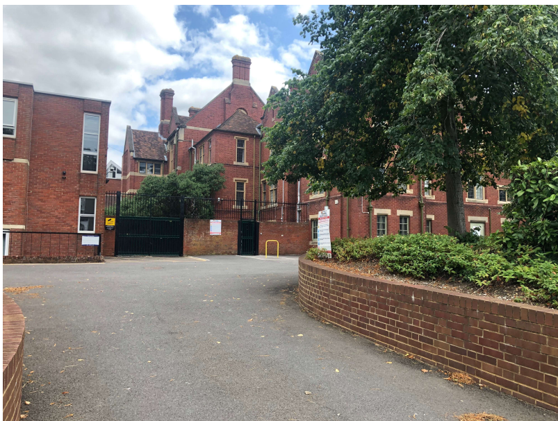
Fig 2- Access road from Redlands Road
