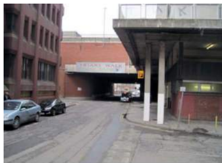
Garrard Street and Friars Walk Car Park
