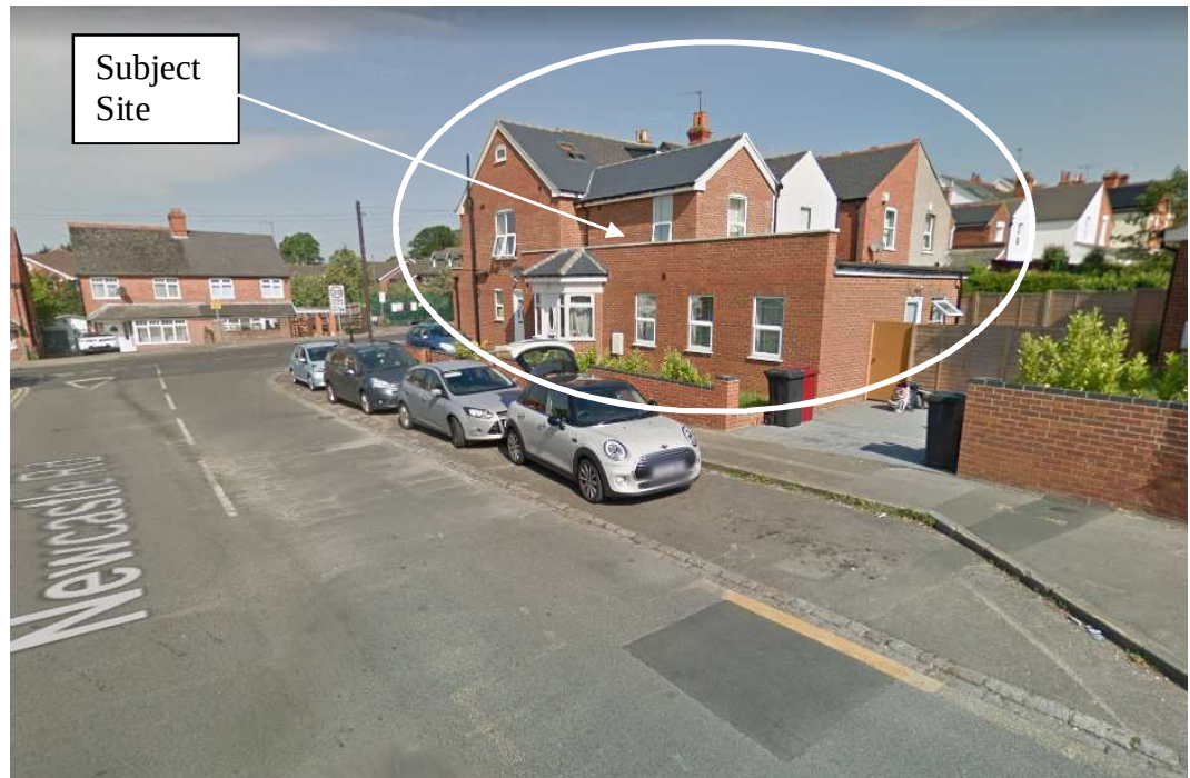
Figure 3: Newcastle Road looking west – View of subject site frontage
