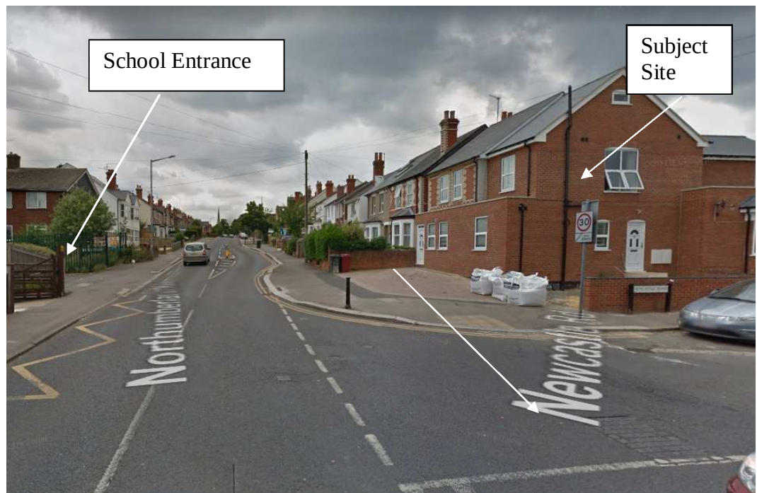
Figure 4: Northumberland Avenue looking north - view of subject site frontage
