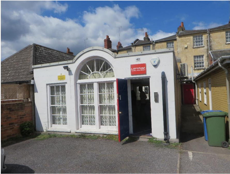
Rear extension seen from parking area
