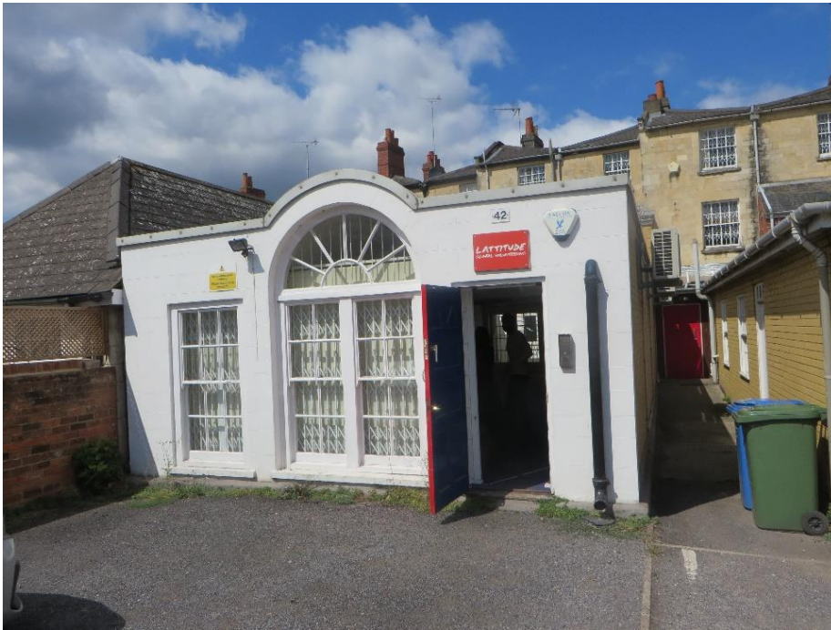
Rendered rear elevation of modern extension
