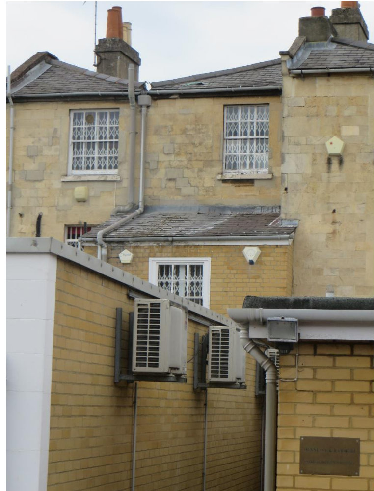
Modern extensions (in yellow brick) to rear at ground and first floor levels
