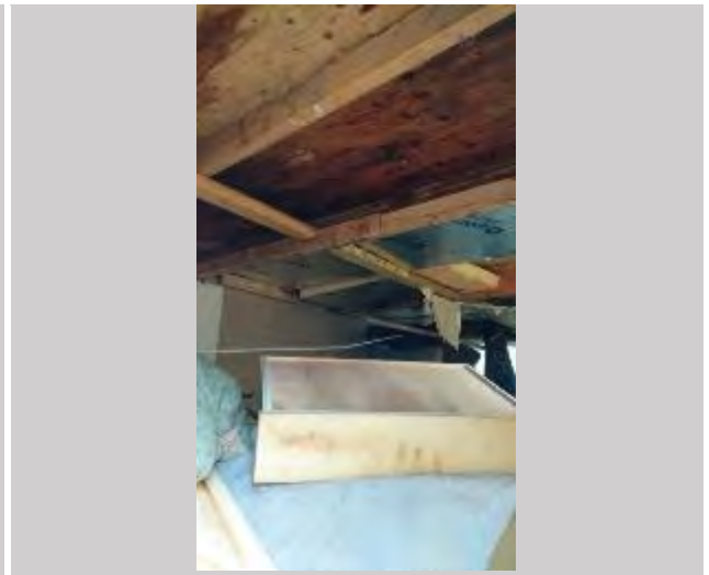
Photograph 12: Building 2 – internal view facing northwest.
