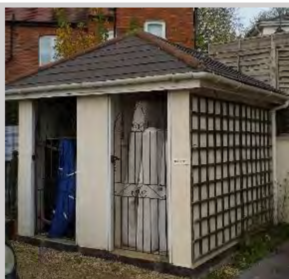
Photograph 6: Building 4 – east and south elevations.
