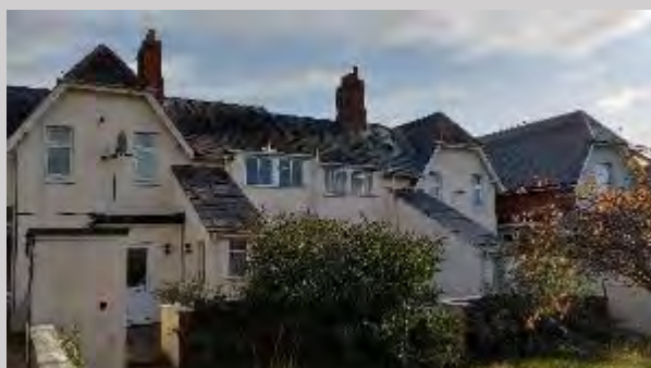
Photograph 1: Building 1, Sections A and B – west elevation.
