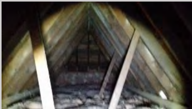
Photograph 9: Building 1 – loft space in Section C facing east.
