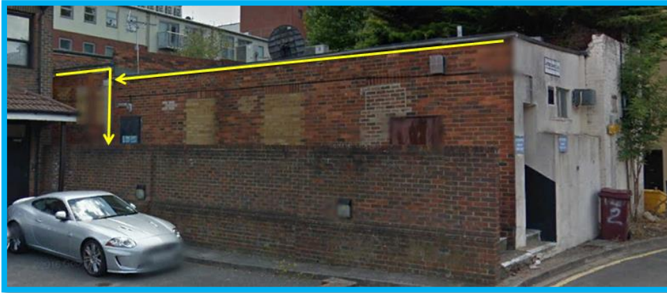
Fig 6 Existing rainwater drainage for the west of the site (Google Street View).
