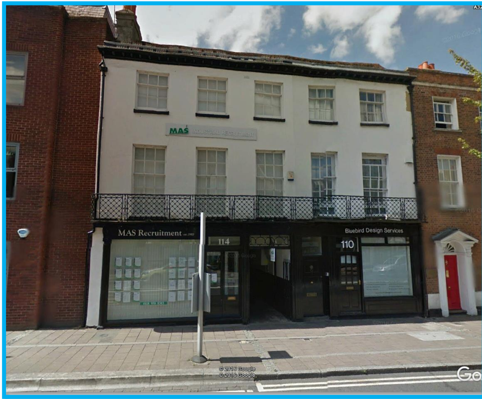
East entrance to 112 London Street (Google Streetview)
