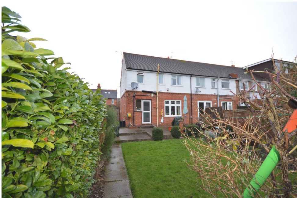
Rear elevation, indicating steps and patio down to lawn.
