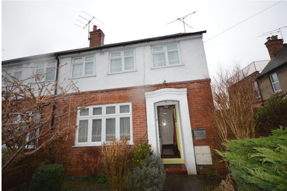
Front Elevation indicating the current threshold at approx..300mm from ground level (over 4 bricks high)
