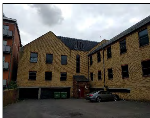
Figure 4: Eastern and northern elevations of building
