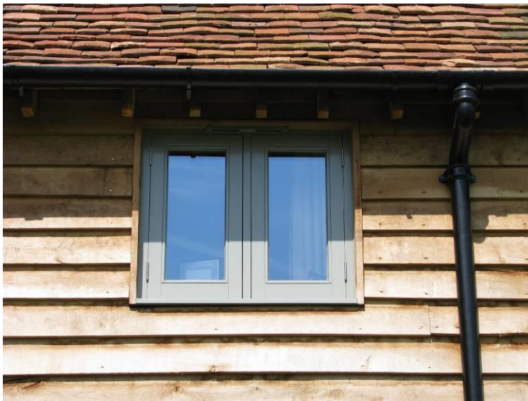
Figure 17: Examples of Conservation flush casement window and metal (cast iron) rainwater goods.
