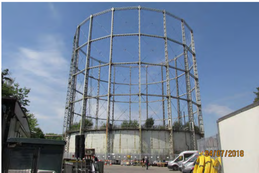
Plate 2. Gasholder located within the site
