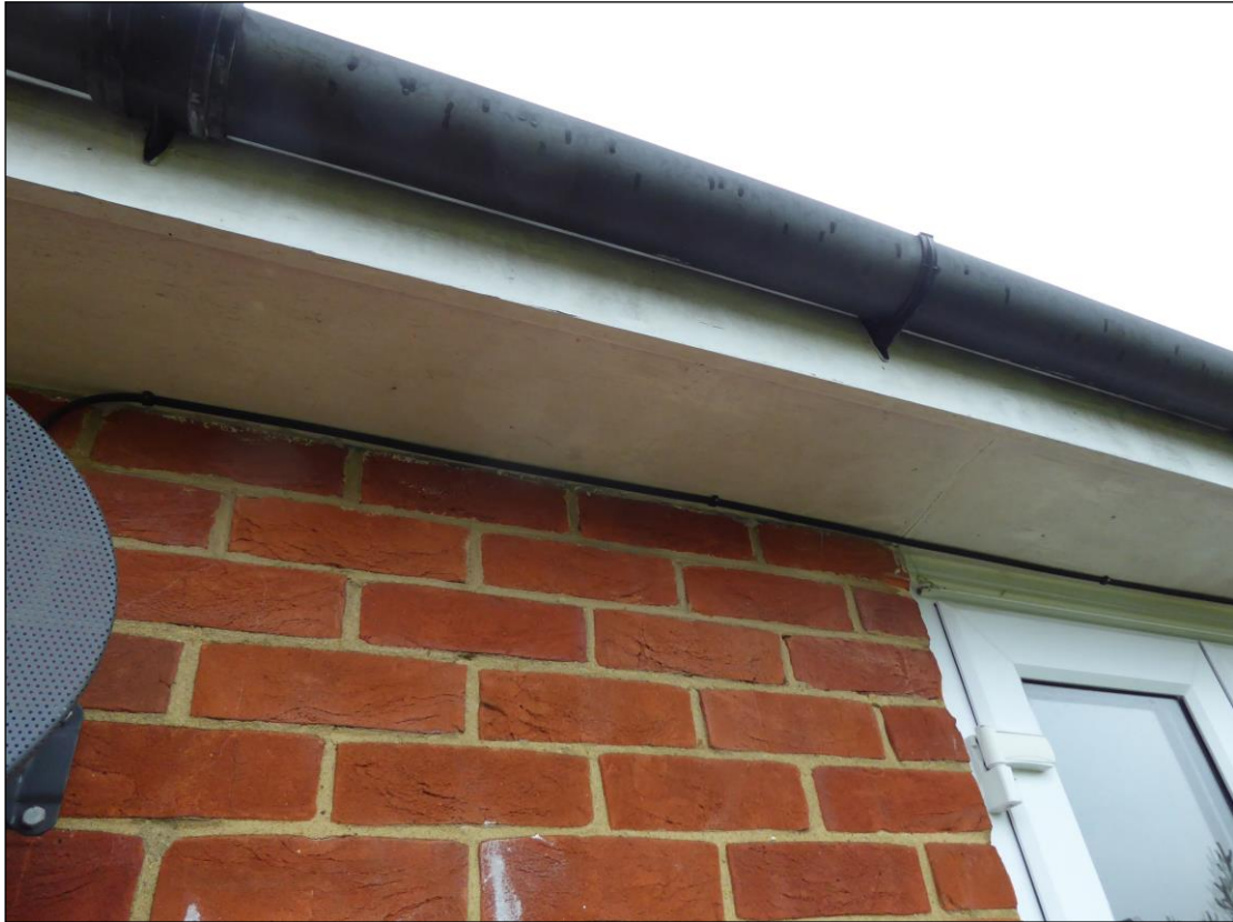
Figure 6. Example of soffits, 4 Highdown Avenue, Emmer Green 09.04.18
