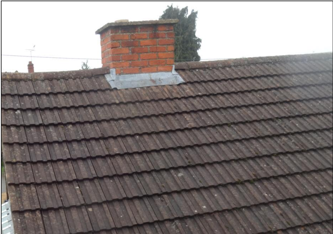
Figure 5. Ridge tiles and chimney flashing, 4 Highdown Avenue, Emmer Green 09.04.18
