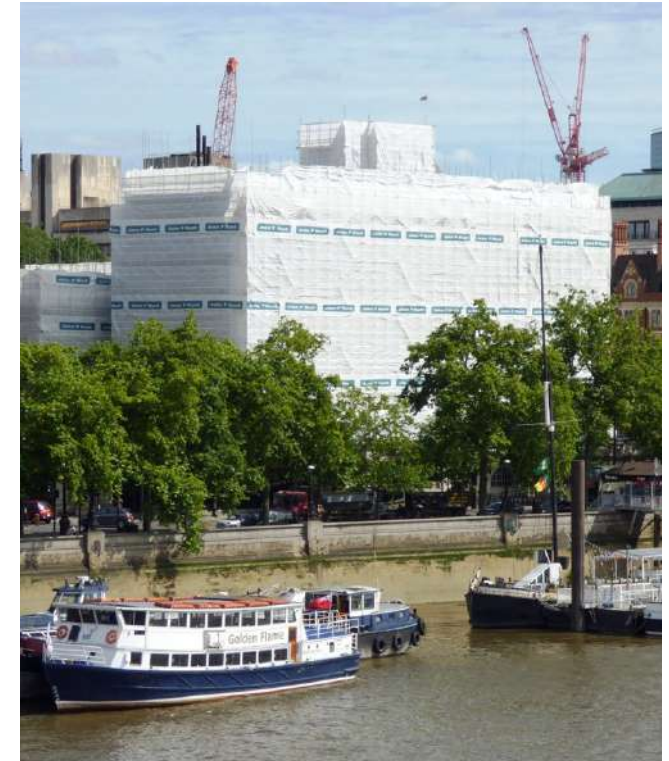
Example monarflex sheeting on another inner-city site, used to contain dust, noise and emissions protecting arboriculture.
