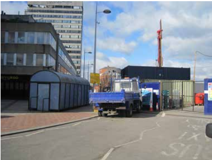
Plate 2: Station improvement works being carried out on Station Hill to the north of the Site.
