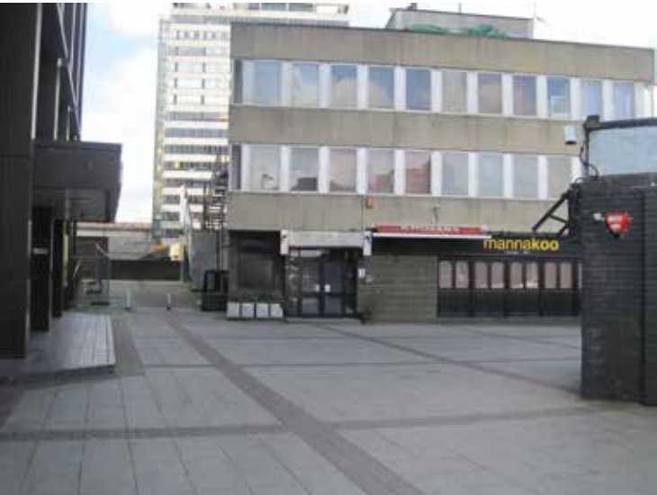
Plate 4: View westwards towards the three storey building.
