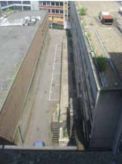
Plate 16: View northwards along the western exterior of Telecom House (pictured right) from the 7th floor of the Friar Street block.
