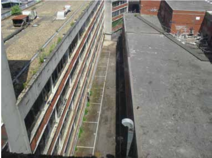
Plate 15: View northwards along the eastern exterior of Telecom House (pictured left) from the 7th floor of the Friar Street block.
