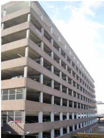
Plate 12: Multistorey Car Park.
