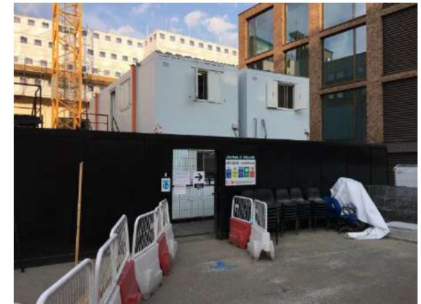
Above: Example welfare entry with cabins, hoarding and segregated pedestrian route
