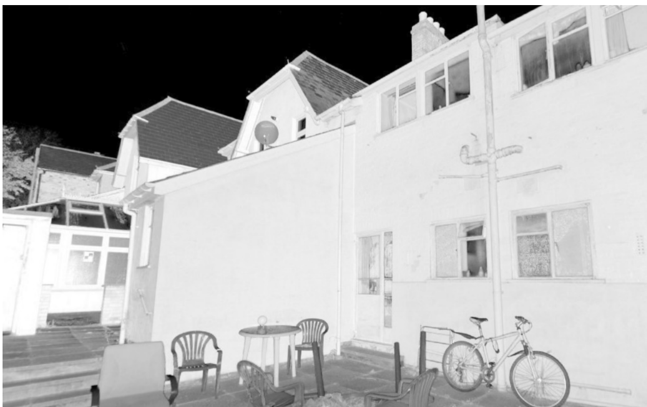
Figure 5 Rear patio as existing
