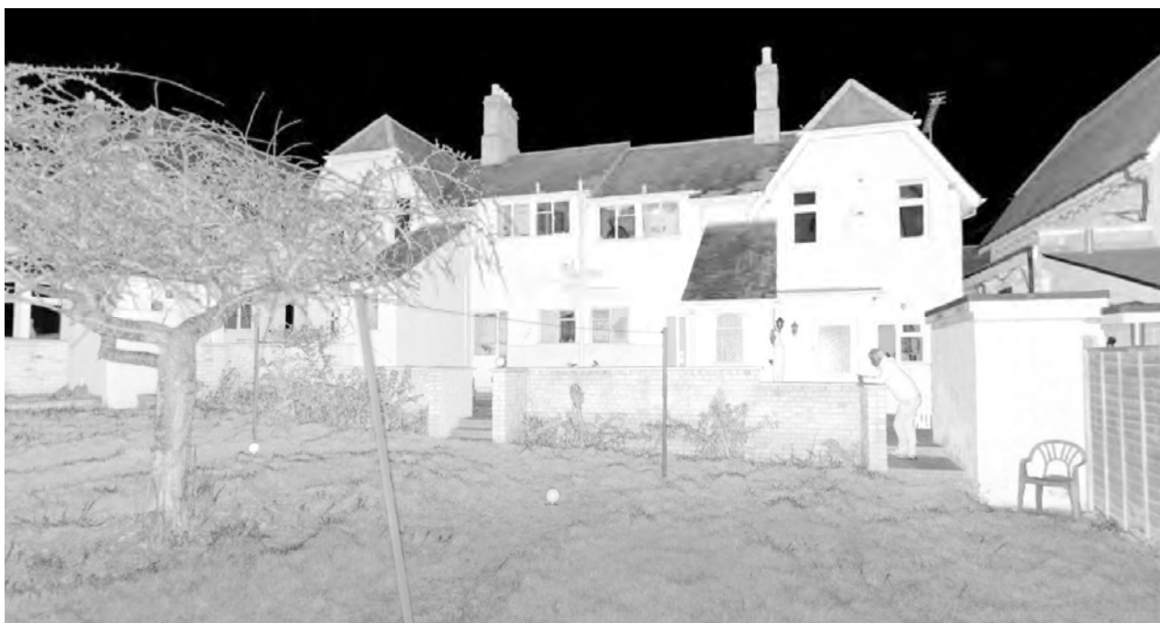
Figure 4 Screenshot of the 3D survey model: the rear of the building
