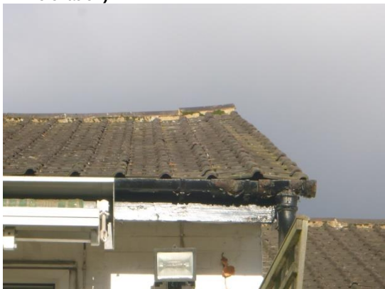
5. Ridge tiles tightly fitted with mortar intact (rear elevation).
