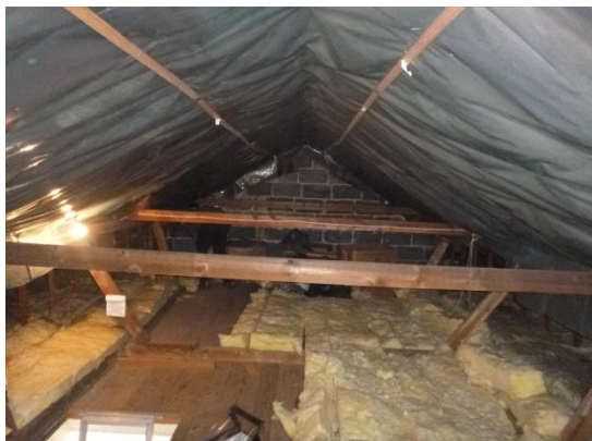
13. Eastern section of roof void viewed from the old external wall.
