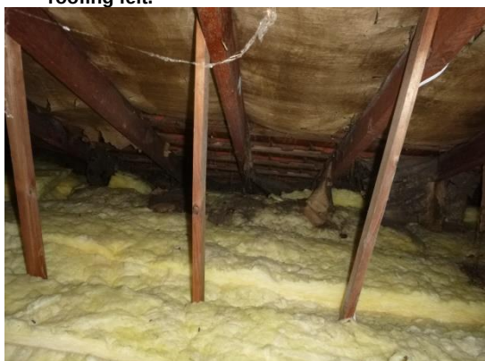
17. Fibreglass insulation in the western section of roof void.
