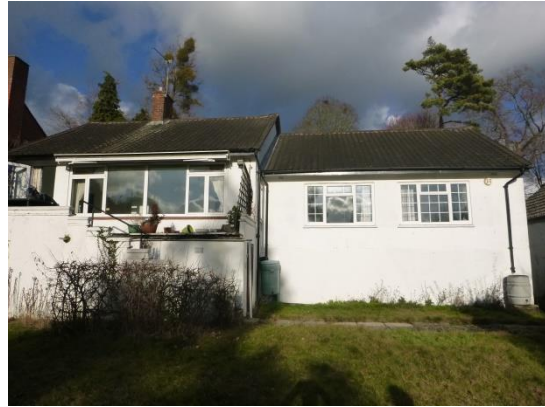
2. Rear of the bungalow viewed from the southwest.
