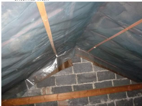
15. Plastic sheeting covering the old bitumen style roofing felt.
