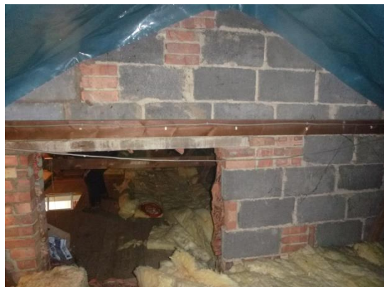
14. Old external wall in the centre of the roof void.
