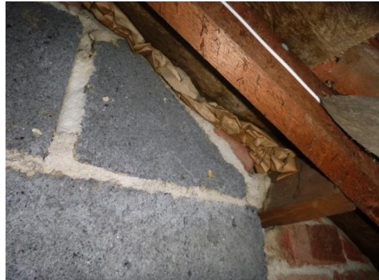
22. Edge of wall behind timber rafters insulated with paper.
