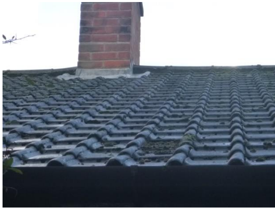
7. Lead flashing tight around chimney (front elevation).
