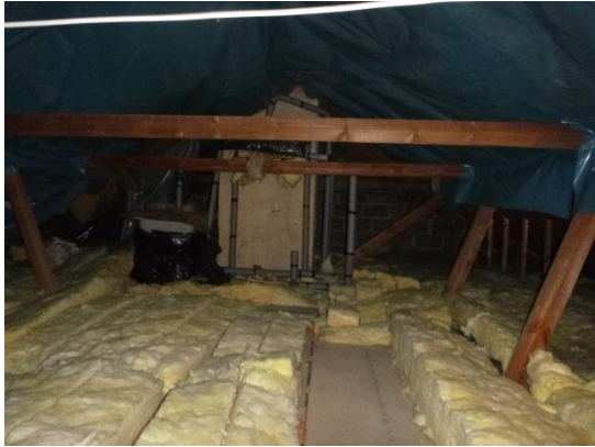
19. Chimney in the western section of the roof void with two water tanks.
