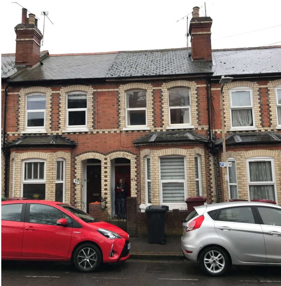
Front elevational view of 41 Field Road
