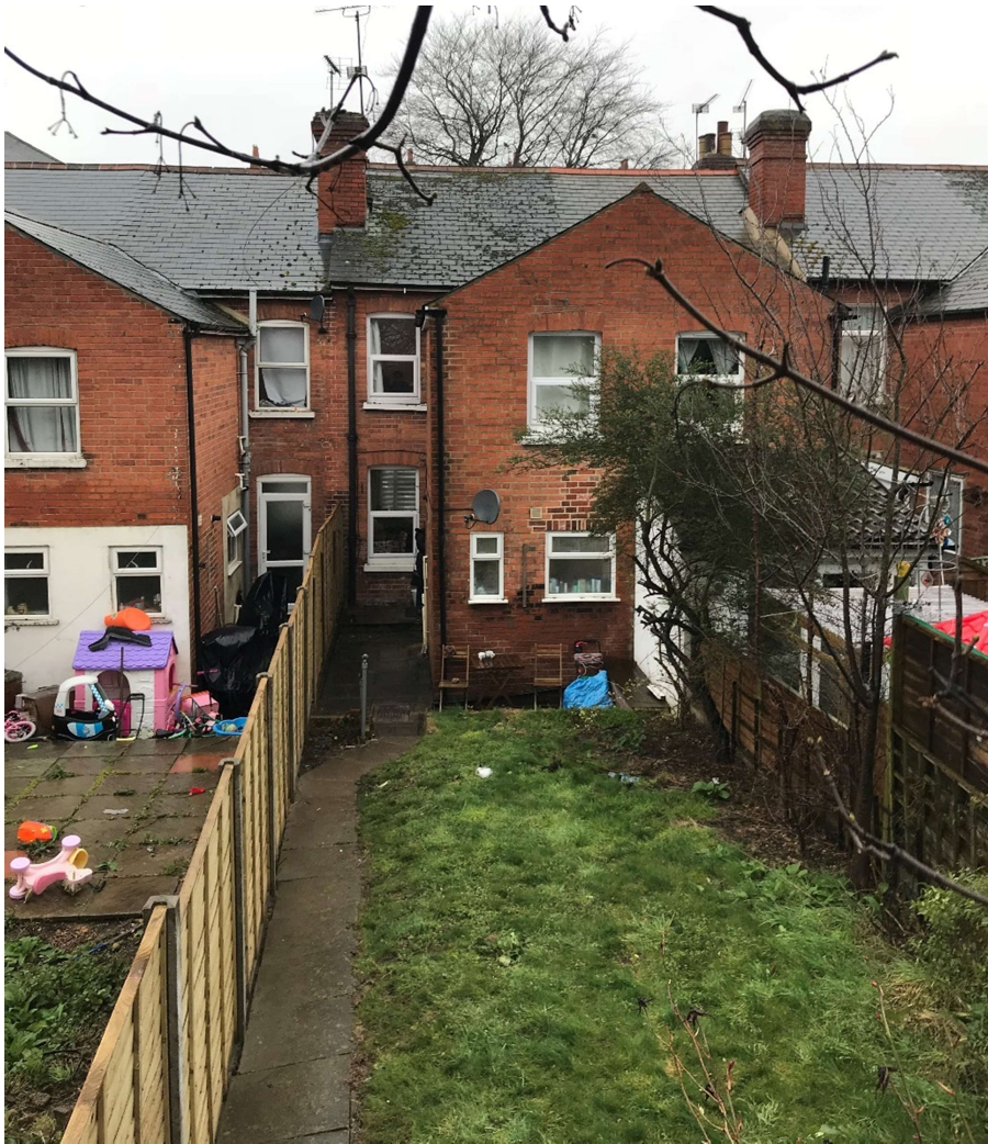
Existing rear view of 41 Field Road, showing the existing extension to the adjoining neighbour at no. 39
