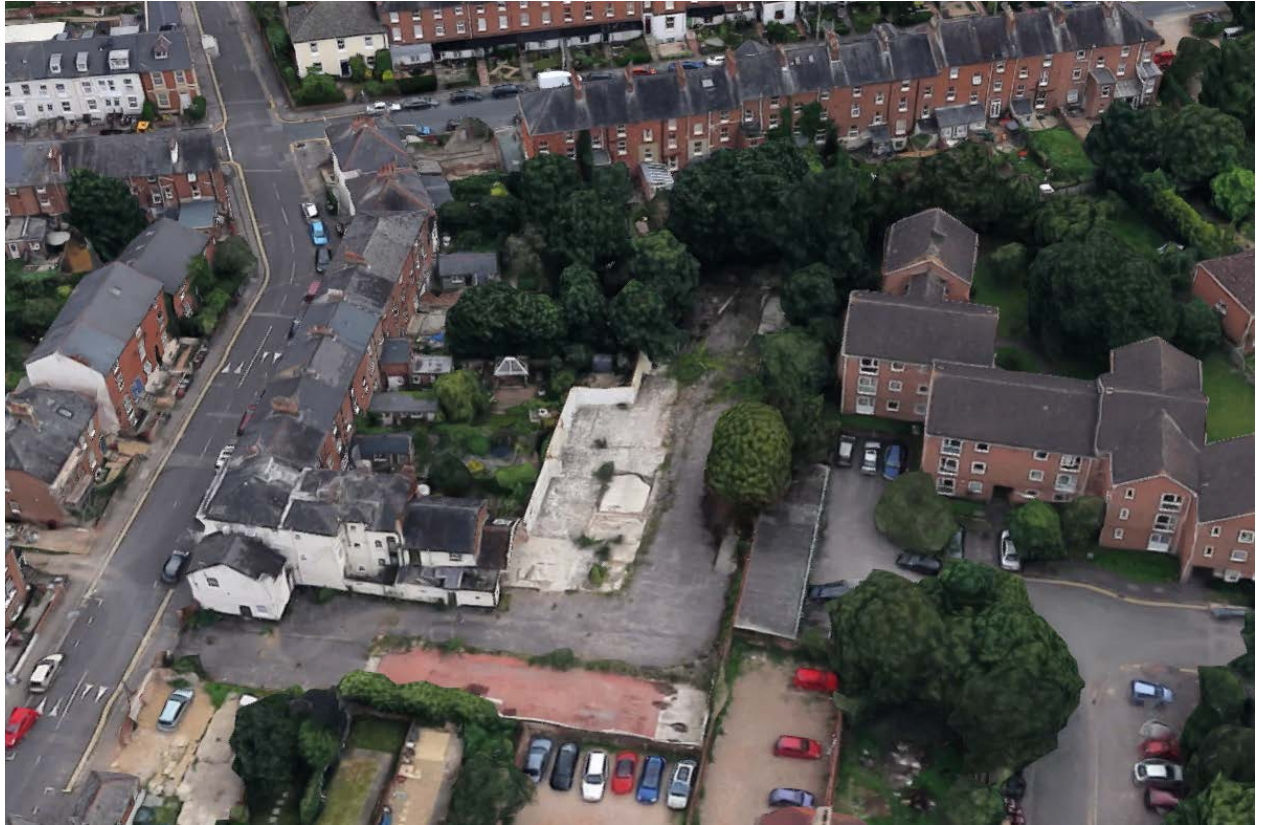
Aerial view looking east
