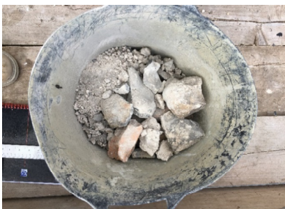
Three separate façade opening up areas all with rubble wall to full depth behind.
