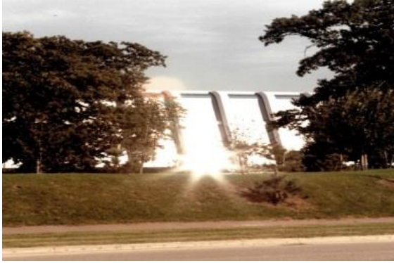
Solar glare on a sloping facade
