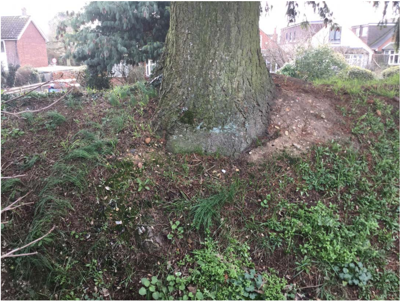
SAL8 Base of tree on ridge of embankment.
