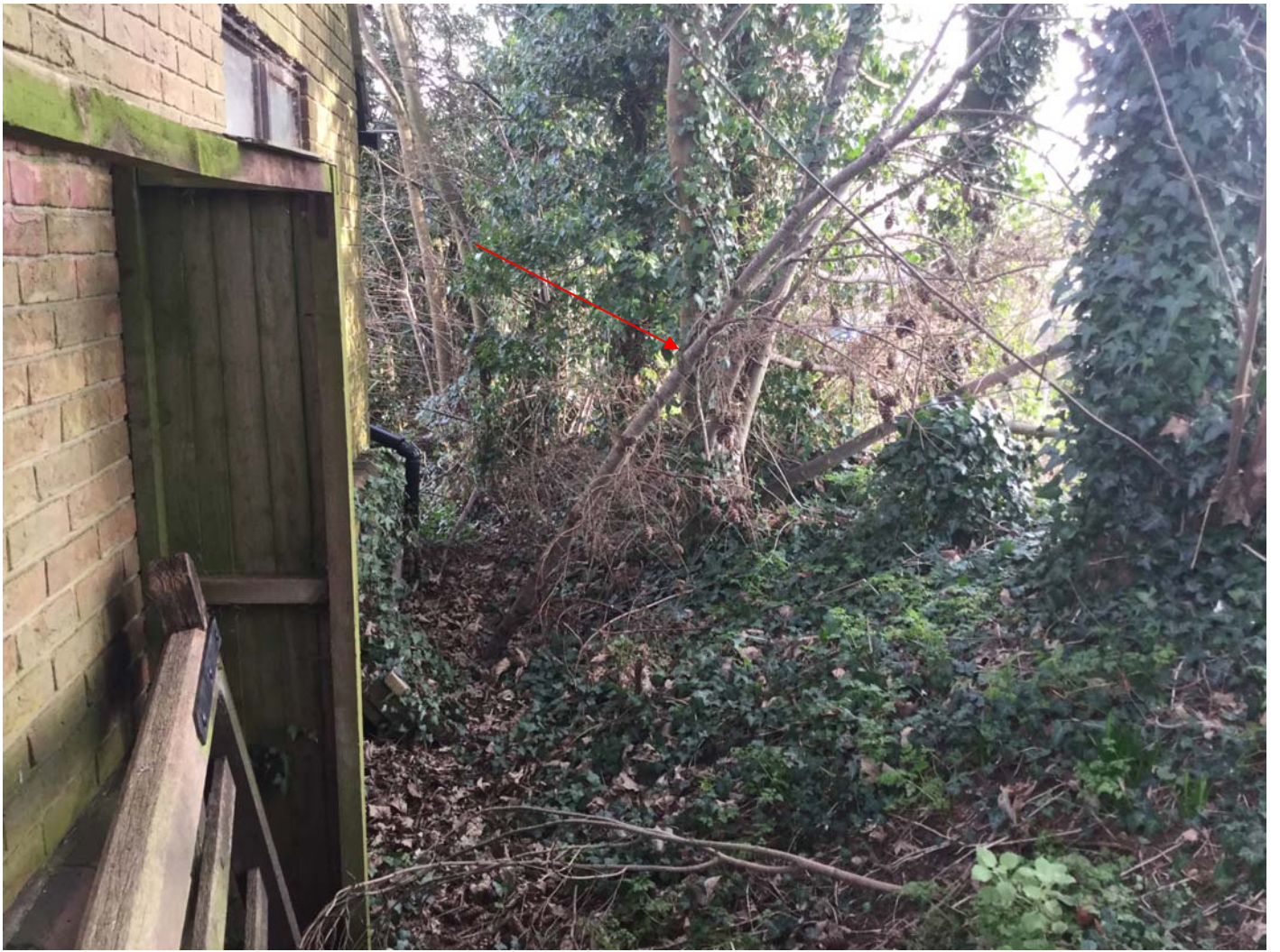
SAL4 Historic branch failure identified by red arrow.
