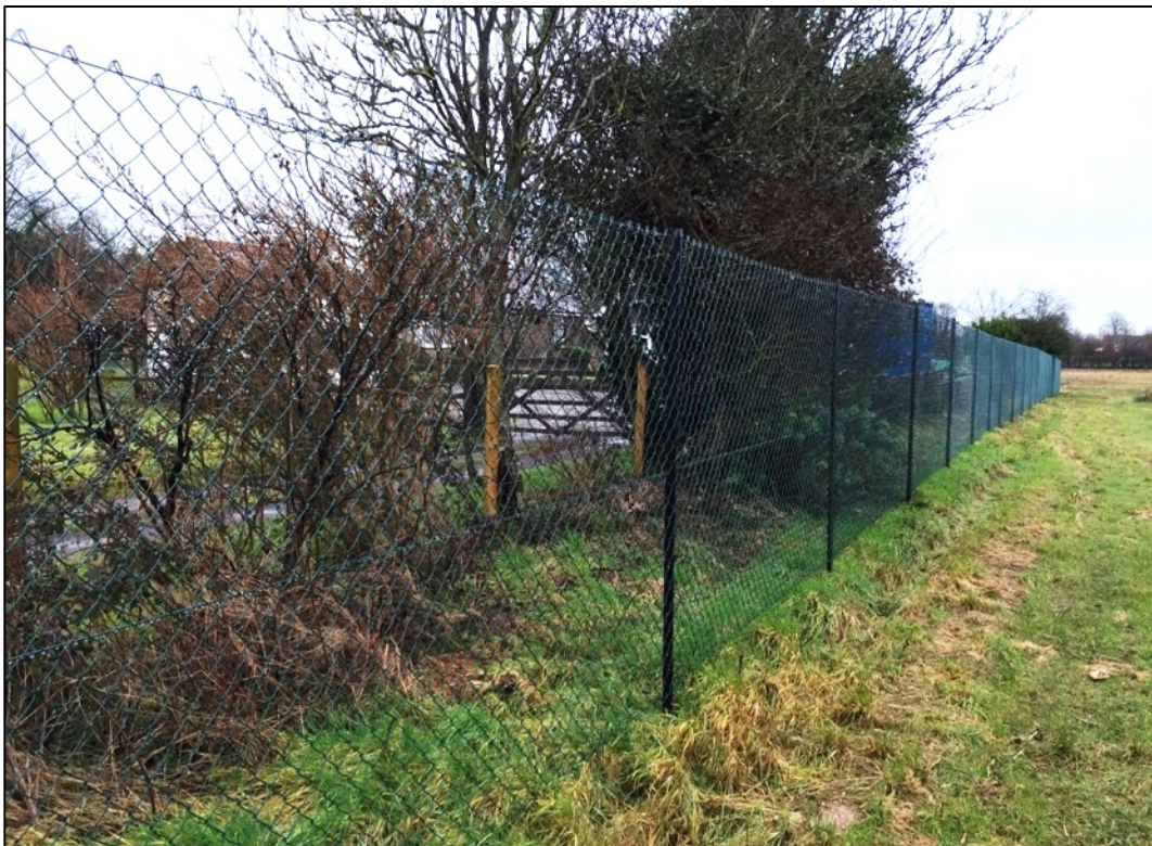
Chain-link on angle-iron uprights
