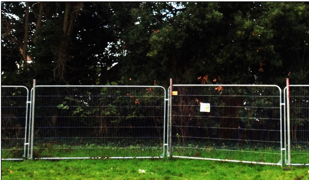
Weld-mesh panels on scaffold uprights
