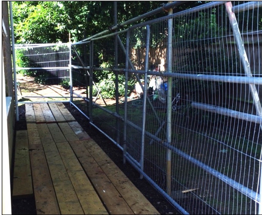
Scaffold board pedestrian ground protection
