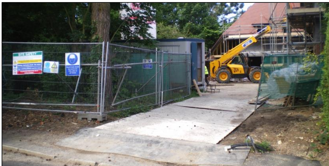
Vehicular ground protection trackway
