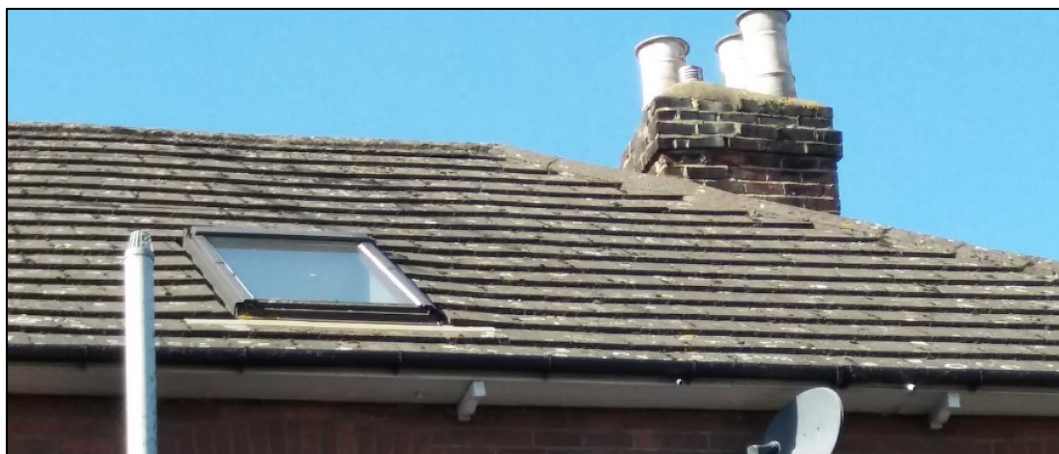
Figure 9 – roof showing good condition of main and ridge tiles
