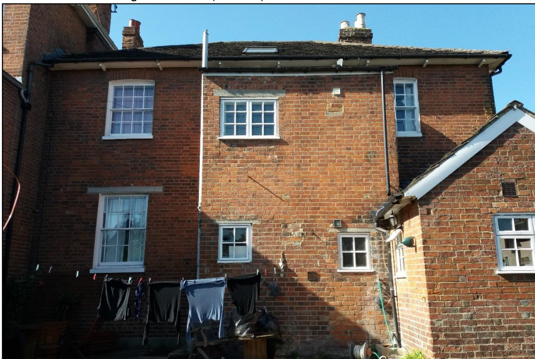
Figure 3 – Rear (eastern) elevation of 1 Jesse Terrace
