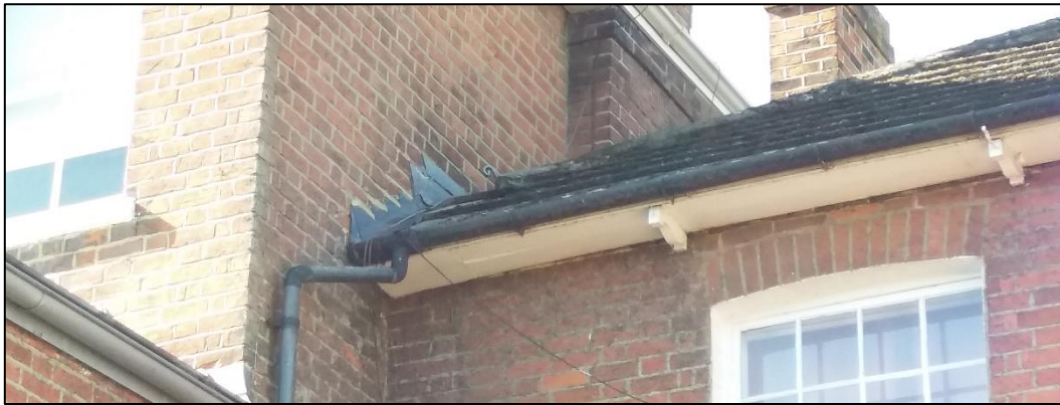
Figure 11 – roof tiles, boxed eaves and flashing between the two buildings
