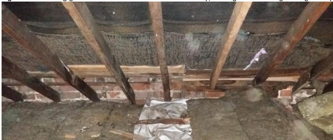
Figure 8 – showing the wall-plate extending into the roof void, separating roof and eaves
