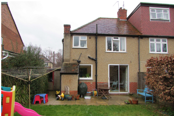
Rear elevation no. 23 Geoffreyson Road.
