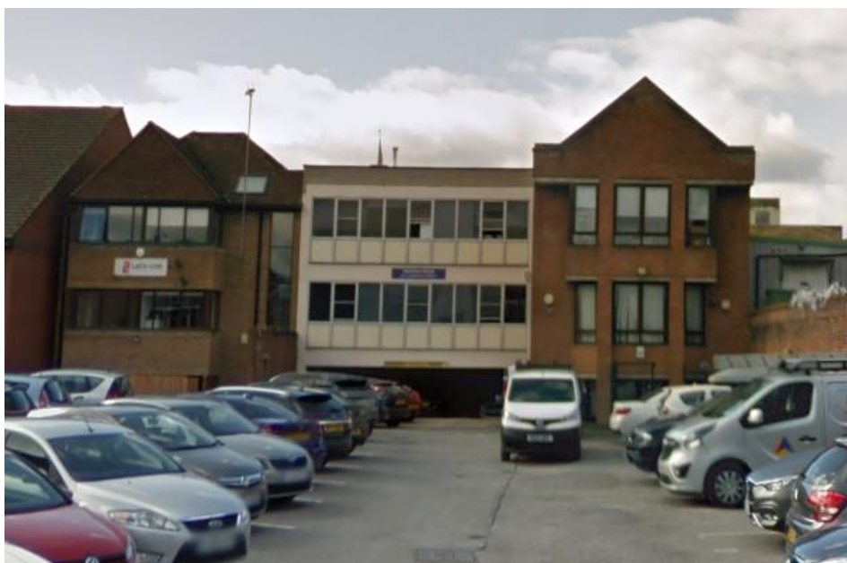
View of Rear Elevation
