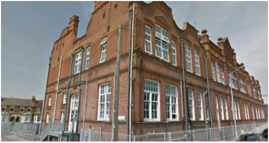
E.P. Collier Primary School is a substantial period building to the north of the development site. Materials are of traditional "Reading Red" brick construction with an increased level of brick detailing typical of landmark institutional buildings in the local area.
