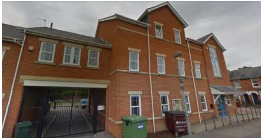
The New Hope Centre is a recent 2½ - 3 storey development comprising a collection of townhouses and apartments.
