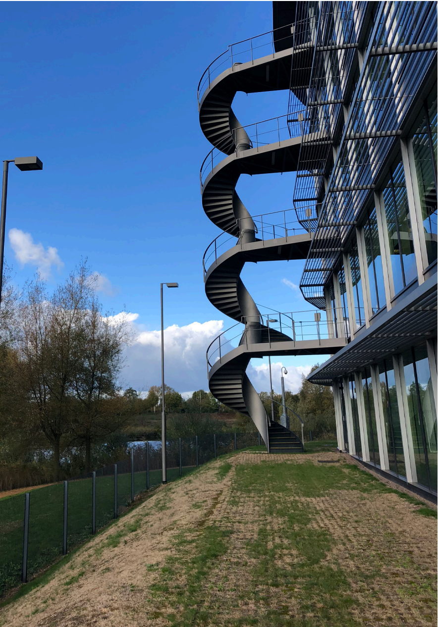
EXISTING ROUTE FROM THE FIRE ESCAPE STAIR OVER UNEVEN PAVING
