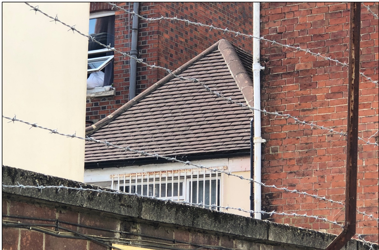
Photograph 2. The hipped roof of 43 London Street's eastern aspect.
