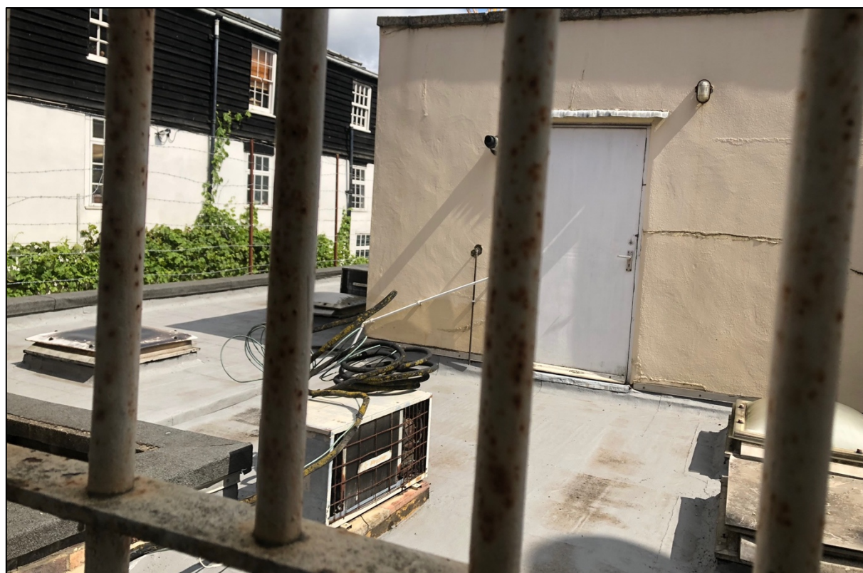
Photograph 4. Flat-roof sections of 43A London Street.
