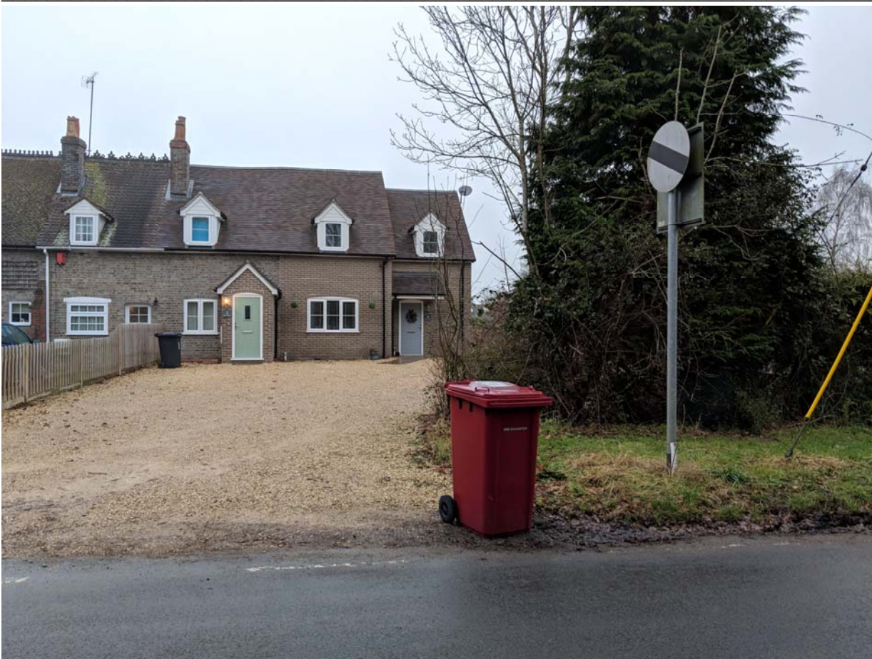
Figure 2-10: No. 2 and No. 3 Kiln Cottages, View from Kiln Road (Prior construction of 3a Kiln cottages)
