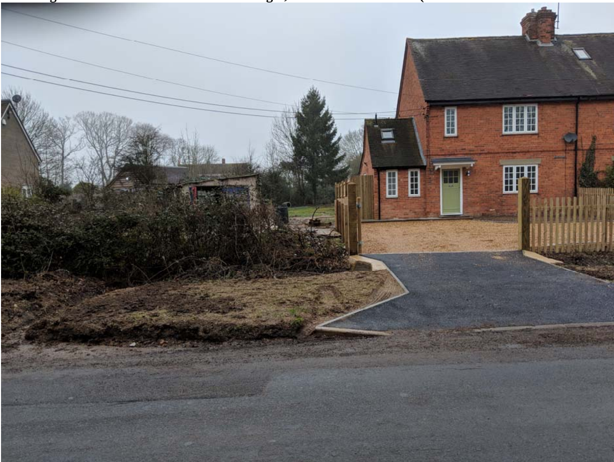
Figure 2-11: No. 2 Felix Cottages, View from Kiln Road
