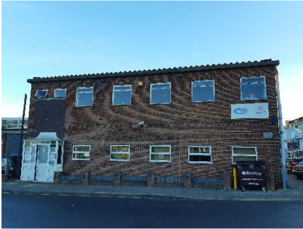
Photograph 1. The western elevation of 16 North Street, Reading.
