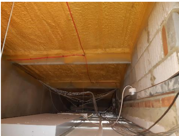
Photograph 5. The roof space.
