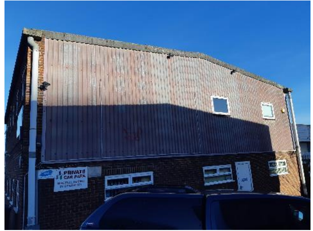
Photograph 2. The southern elevation of the building.
