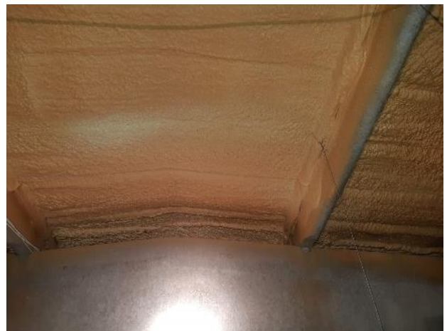
Photograph 6. Detail of the underside of the roof.
