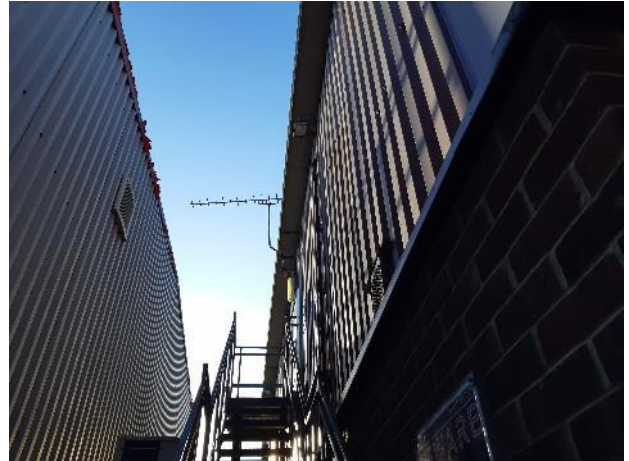
Photograph 4. The rear (eastern) elevation of the building (to the right side of the photograph).
