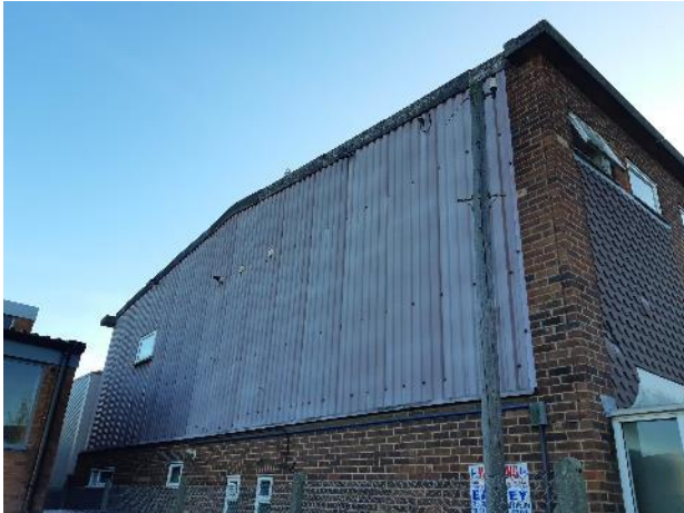
Photograph 3. The northern elevation of the building.
