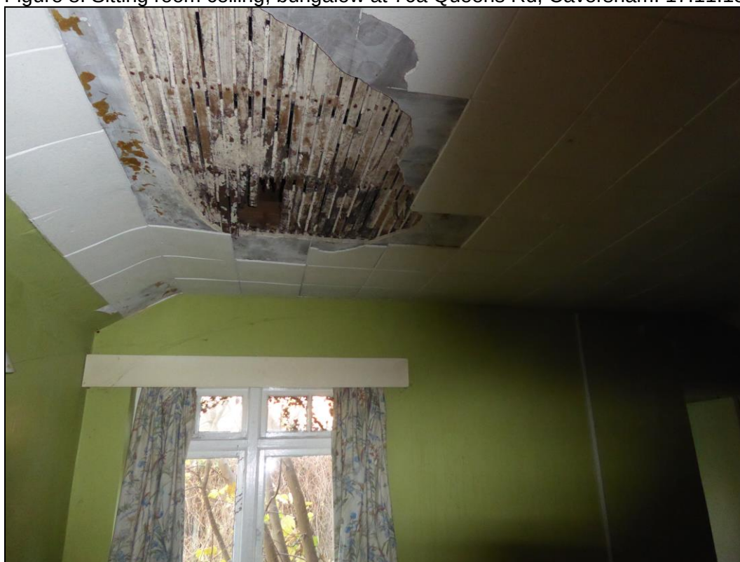
Figure 8. Sitting room ceiling, bungalow at 76a Queens Rd, Caversham. 17.11.18
