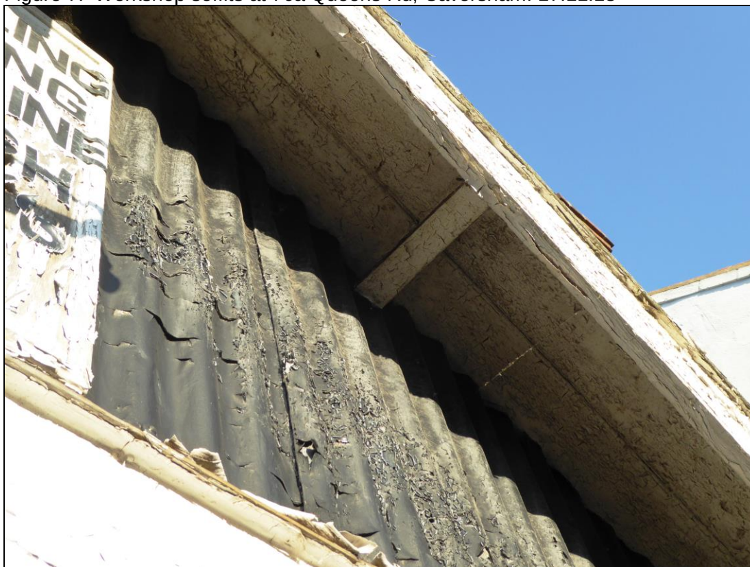
Figure 7. Workshop soffits at 76a Queens Rd, Caversham. 17.11.18
