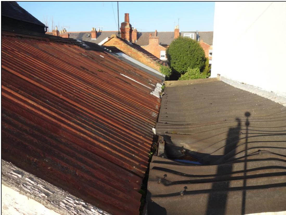
Figure 3. Workshop roof and covered passageway to the east, 76a Queens Rd, Caversham. 17.11.18
