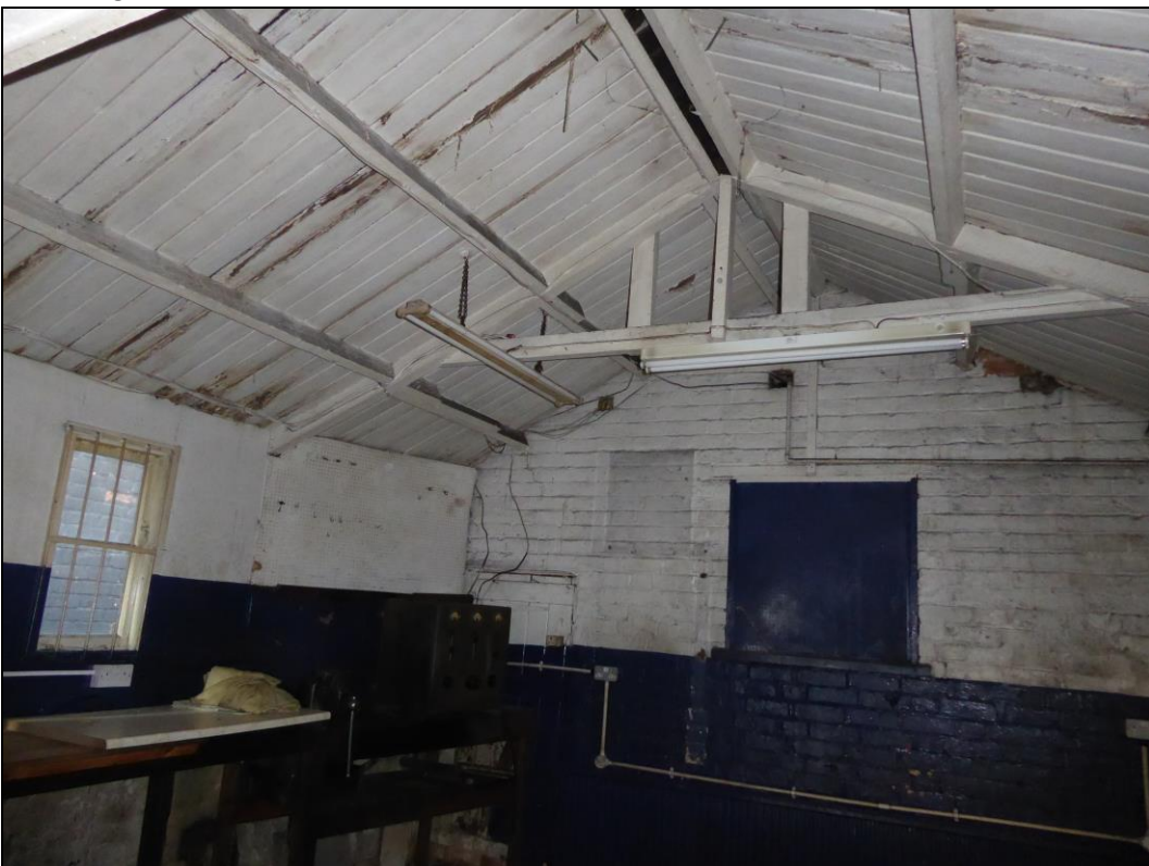
Figure 12. Sarking on the ceiling of the workshop at 76a Queens Rd, Caversham. 17.11.18
