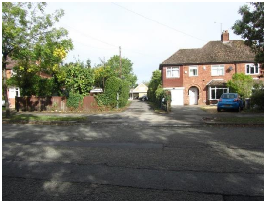
Photo 1: Site Access on The Meadway
