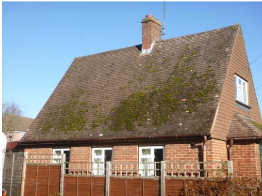
3. Overlapping roof tiles mostly flat, tight and moss-covered (southwest elevation).
