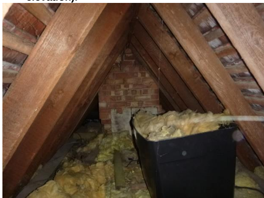
15. Roof void viewed from northwest (rear) gable end.
