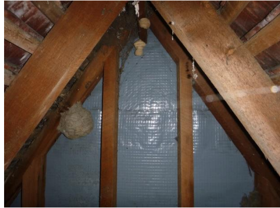
20. Plastic sheeting at gable ends with Celotex insulation behind.
