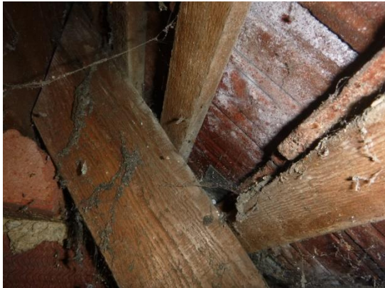
21. Lead flashing visible in roof around chimney.
