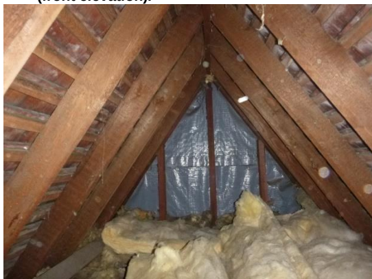
16. Southeast (front) gable end viewed from centre of roof void.
