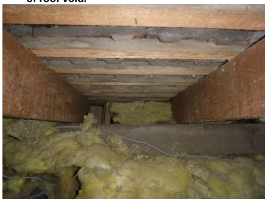
18. Square of fibreglass insulated inside eaves.
