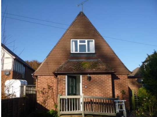
1. Front of the chalet bungalow viewed from the southeast.
