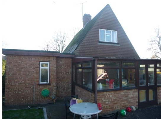
2. Rear of the chalet bungalow viewed from the north.
