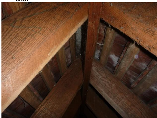
17. Unlined roof with lightly cobwebbed ridge.
