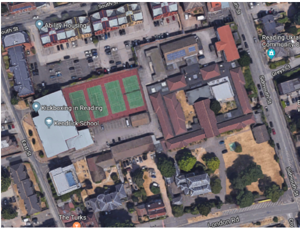
Figure 1 - Kendrick School - Aerial Photo
