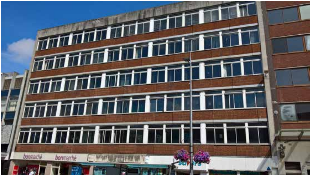
View towards of south of Site from Friar Street
