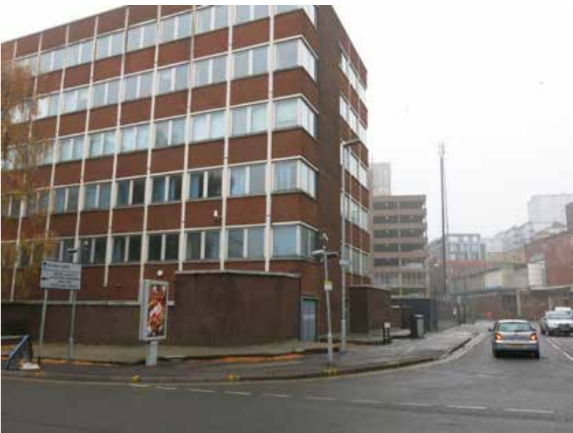
View of the Site from Greyfriars Road
