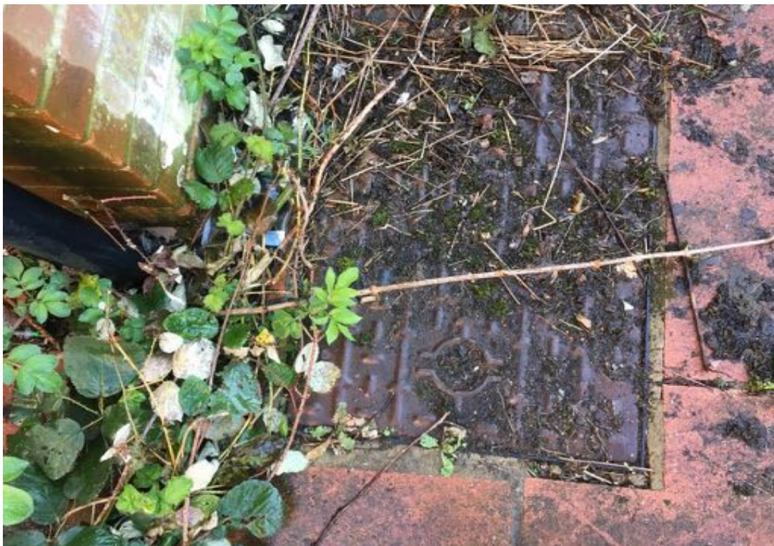
Photograph 18: Assumed drainage manhole located along southern Site boundary
