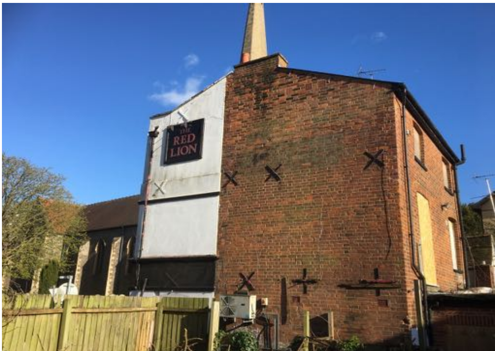
Photograph 4: Side elevation of neighbouring derelict public house positioned directly south of the Site
