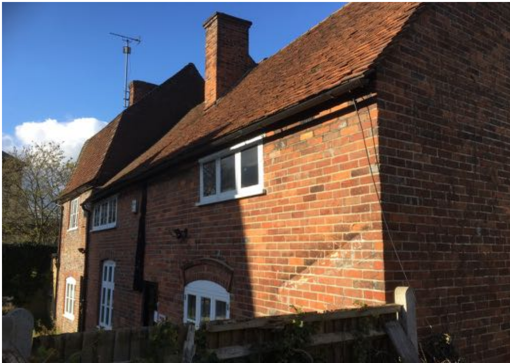
Photograph 5: Rear elevation of neighbouring commercial premises to the north of the Site
